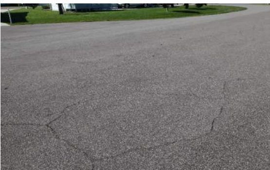
Typical Pavement Condition - Cracking
