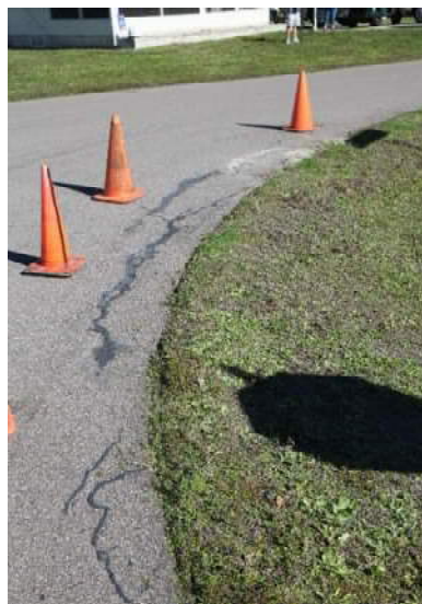
Typical Pavement Condition - Edge Spalling
